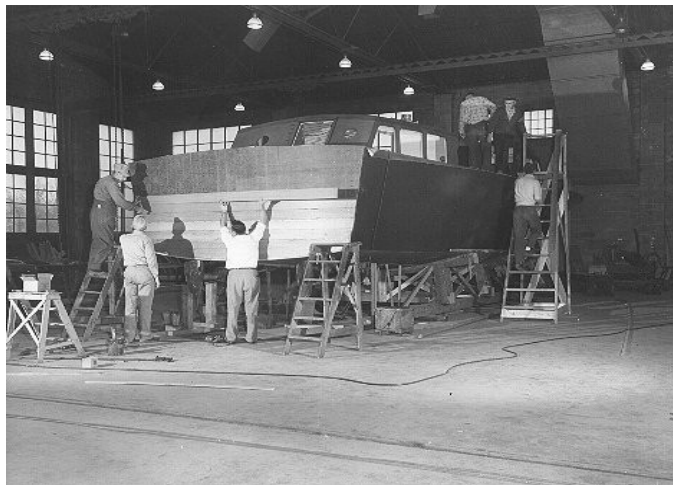
Hacker-built Navy picket boats under construction in 1952
